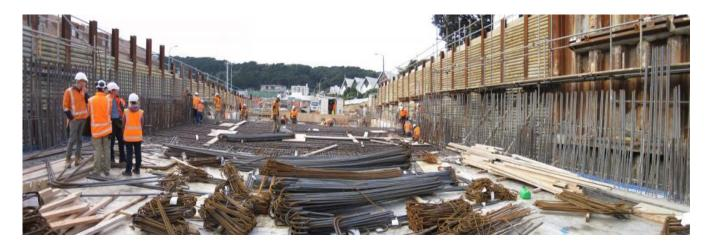
[4]Piles of steel bars lie on the ground ready to be used for more reinforcement in the walls. How does steel reinforcement make the concrete stronger?
