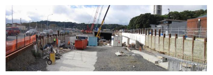
[5]A view from the western end of the trench. Here you can see some of the concrete walls and tunnel roof have been poured. The first roof span to be poured is 14.5 metres wide, 10 metres long and 0.8 metres deep. Can you work out what the total volume of this roof span is in cubic metres?
