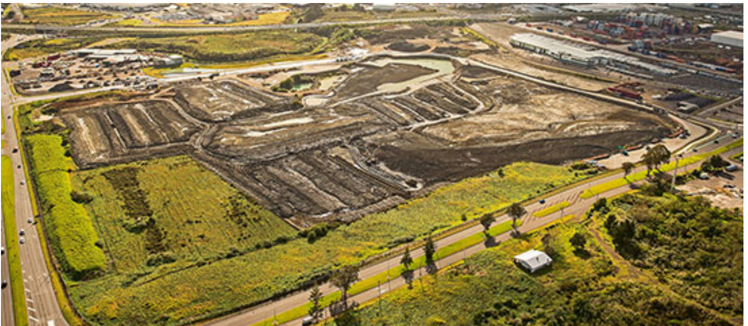
Wiri Quarry: main stockpile (dark grey spoil) and windrows (below reservoir).
